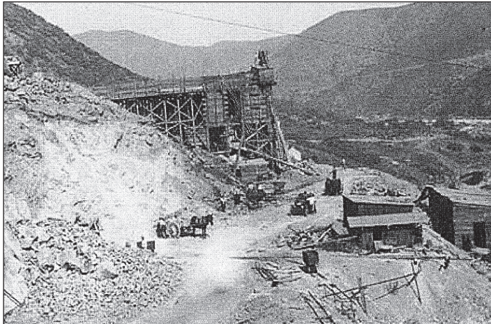
Lake Hodges Dam under construction. July 1917. Courtesy Del Mar Historical Society.
